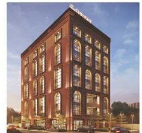
SHRI PARSHVA EMINENT @ ELLISBRIDGE
