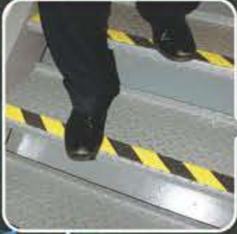
Anti-Skid Staircase System
